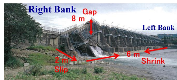
(b) Structural Overview of Shin-Kang Dam (c) Damage Overview of Shin-Kang Dam Fig.5 Topological Relationship of Chelongpu Fault and Shin-Kang Dam and Structural and Damage Overview of Shin-Kang Dam
